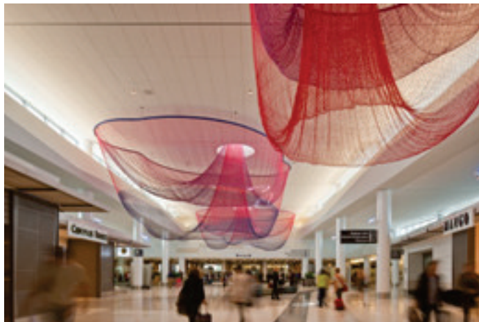
FIGURE 2: Displacement diffusers located in large transit spaces, such as airports, can have a higher face velocity
